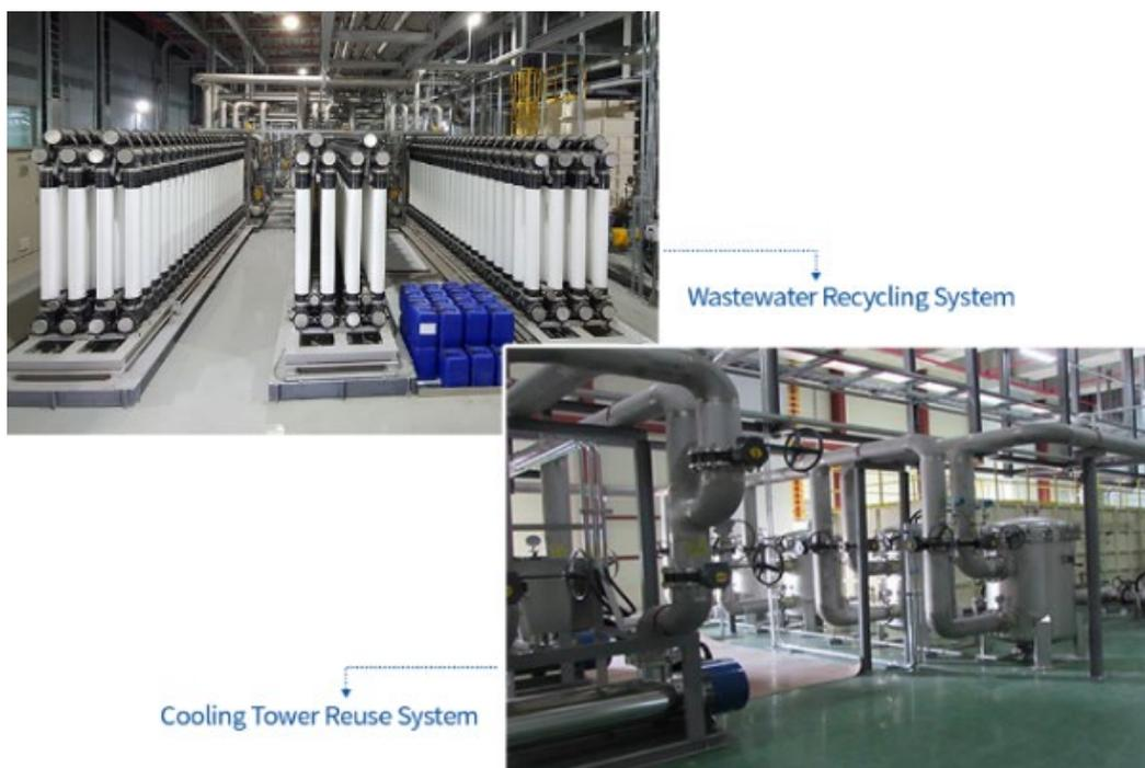
Figure 6: Wastewater Recycling System & Cooling Tower Reuse System of SK hynix
