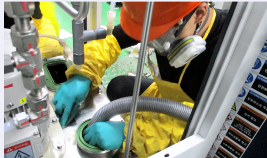
Preventive maintenance work on the inside of scrubber chamber
